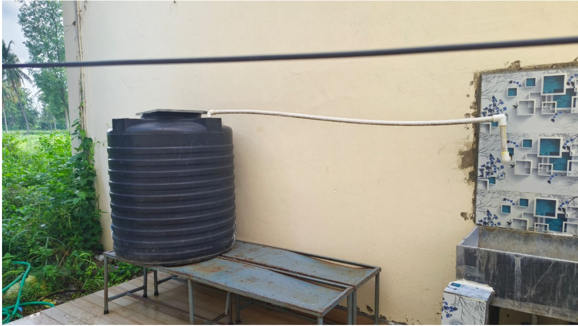
Waste Water Collection from R.O Plant
