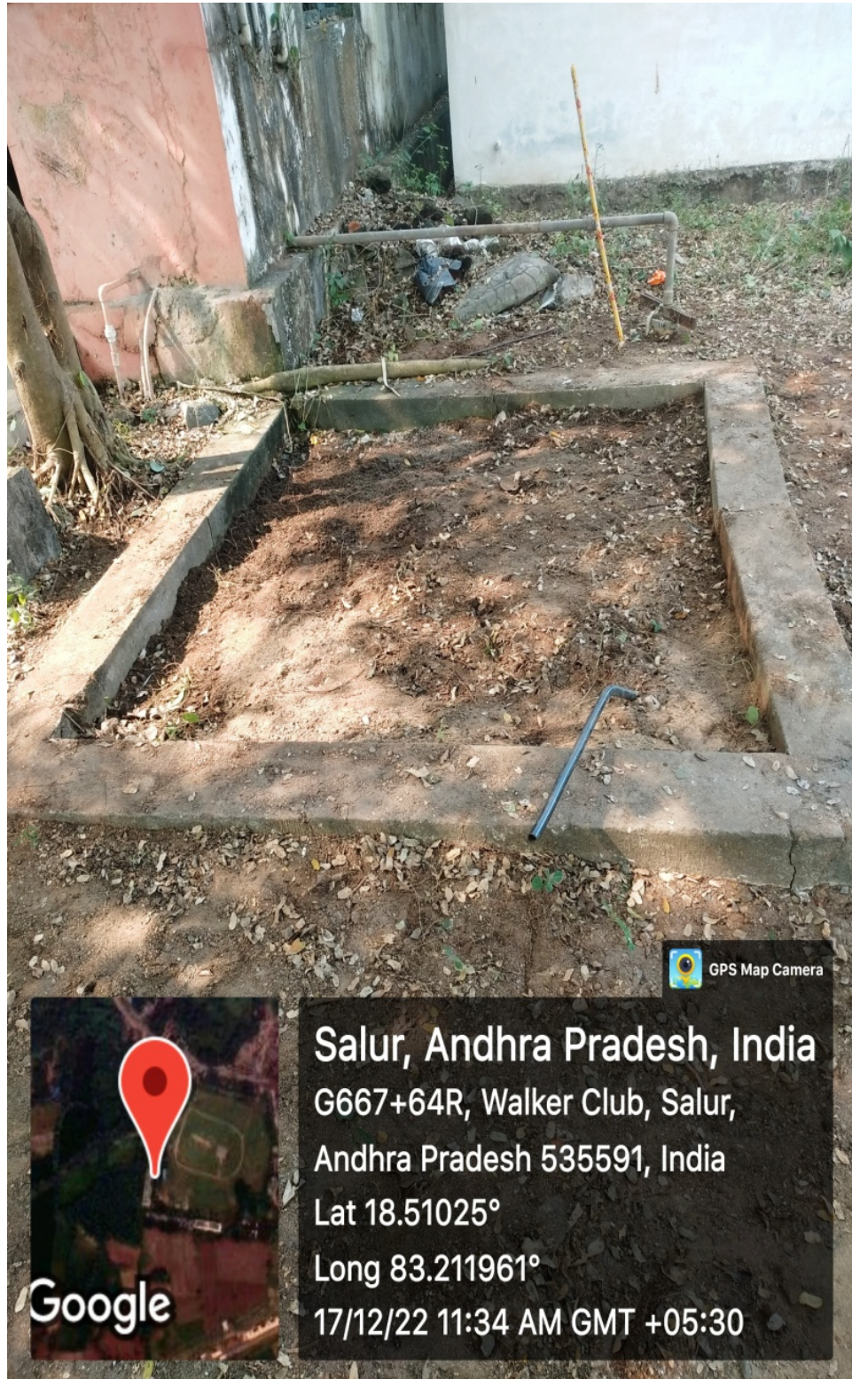
Rain Water Harvesting Soak Pit 1 Near Principal Room (Old Building)
